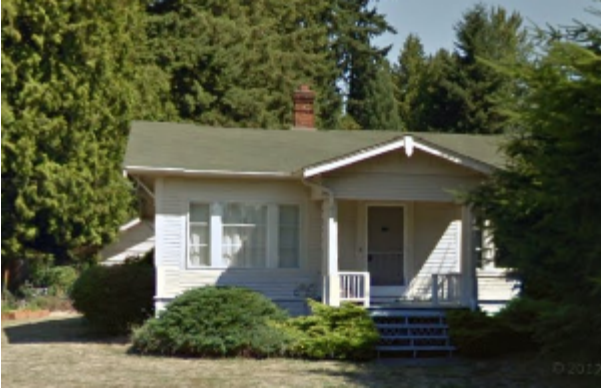
Annabel's house at 11630 NE 90th St. was demolished in 2016
